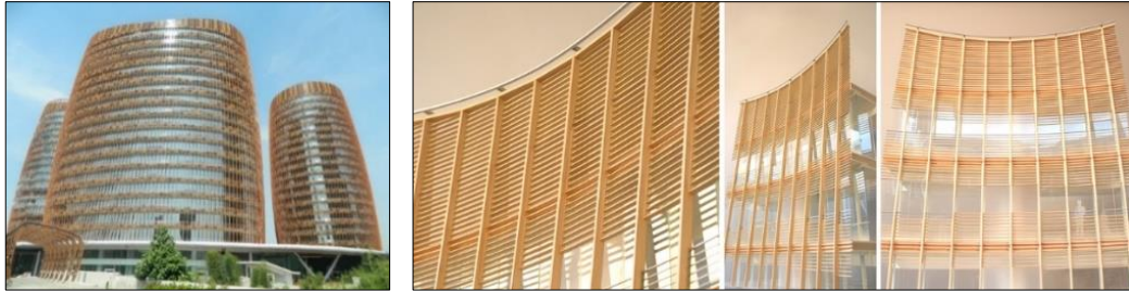
Gambar 1. 1 Gedung Ruang kantor South Quarter dan Desain Fasad Louvre (Sumber: http://dienersyz.com/investments/ dan http://wkkarchitects.com/south-quarter-1/ )
