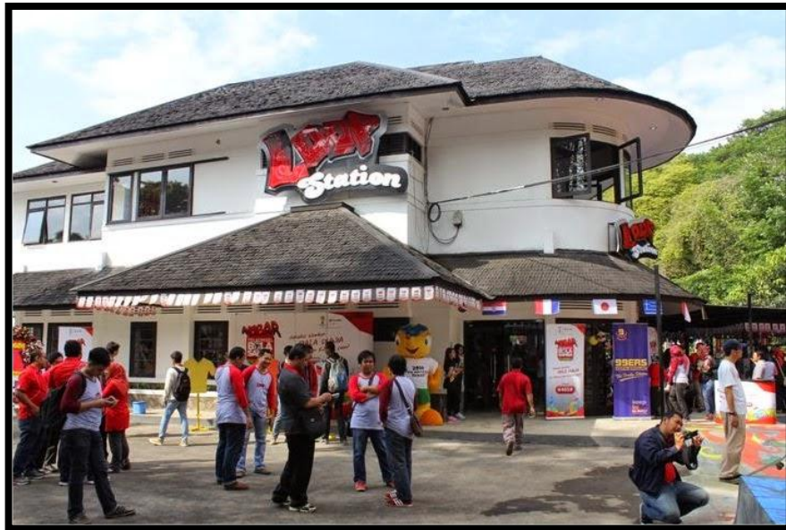
Gambar 5.7 fasilitas loop station
