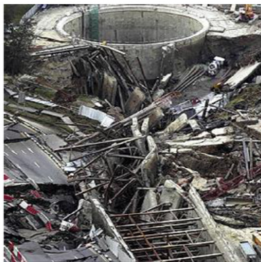
(b). After collapse
