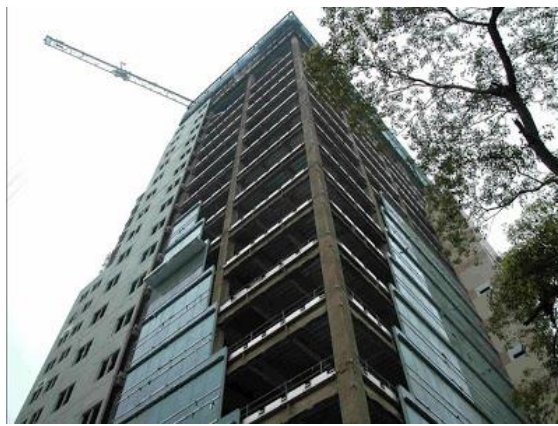
Gambar 1.1 Portal Penahan Momen ( Moment Resisting Frames ), American Institute of Steel Construction
