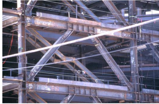
Gambar 1.3 Portal Dengan Pengaku Eksentris ( Eccentrically Braced Frames ), American Institute of Steel Construction
