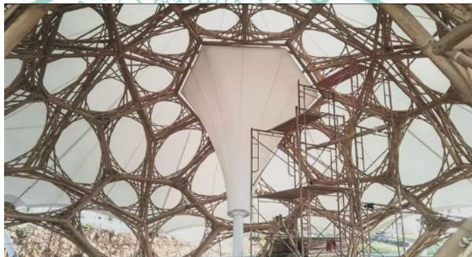
Gambar 1.2 Proses Konstruksi Beachfront Restaurant di Sulawesi Utara Sumber: https://www.instagram.com/p/Ck7HrYMv8il/?utm_source=ig
