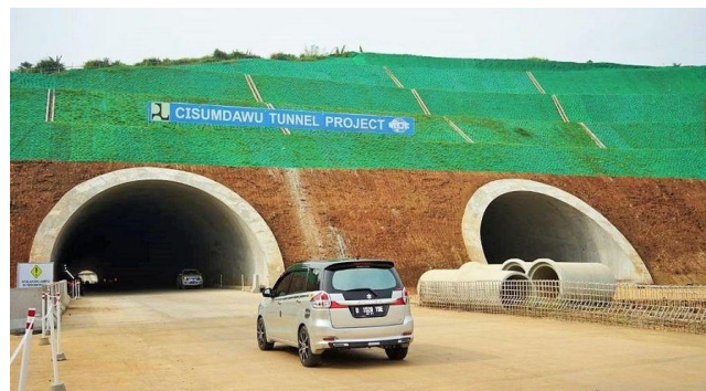
Gambar 1.1. Twin Tunnel Cisumdawu (Pikiran-Rakyat.com, 2020)
