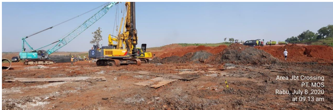
Gambar 1.1 Area Abutmen Jembatan Crossing PT. MOS
