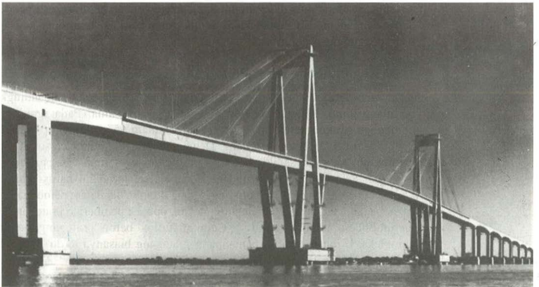
Foto 1.2 Jembatan Chaco-Corrientes, Argentina, jembatan girder boks cable-stayed beton prategang pracetak terpanjang di Amerika Selatan (Atas izin Ammann & Whitney.)
