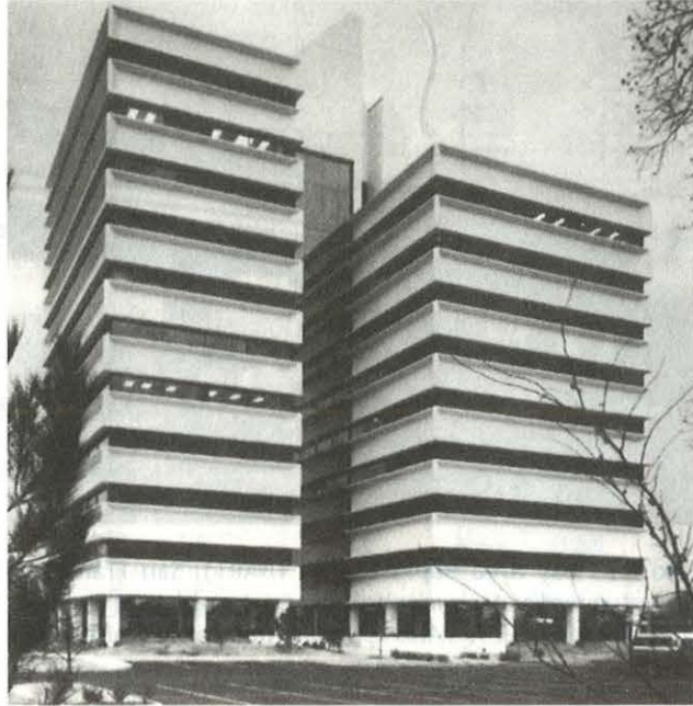
Foto 1.3 Gedung Parkir, Tulsa, Oklahoma. (Atas izin Prestressed Concrete Institute.)
