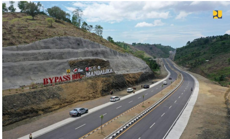
Gambar 3. 1 Jalan bypass Bandara Internasional Lombok – Mandalika
