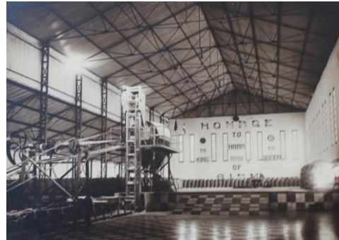
Gambar 1.1 Interior Pabrik Gula Colomadu
