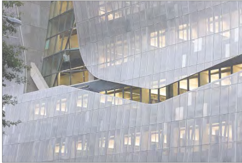
Gambar 1.1. Double skin facade the Cooper Union for the Advancement of Science and Art (Sumber: https://www.archdaily.com/40471/the-cooper-union-for-the-advancement-of-science-and-art-morphosis-architects )
