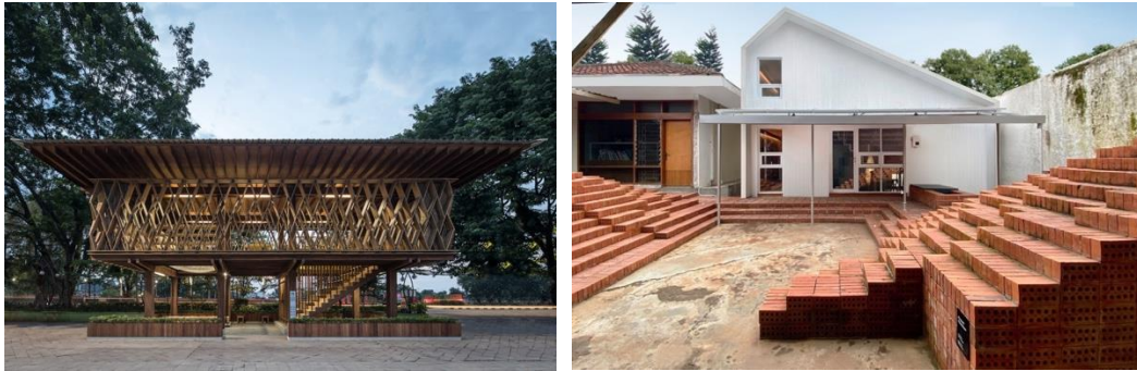
Gambar 1.2 Microlibrary Warak Kayu dan Home-Office Pods AAND Sayana Sumber: Archdaily
