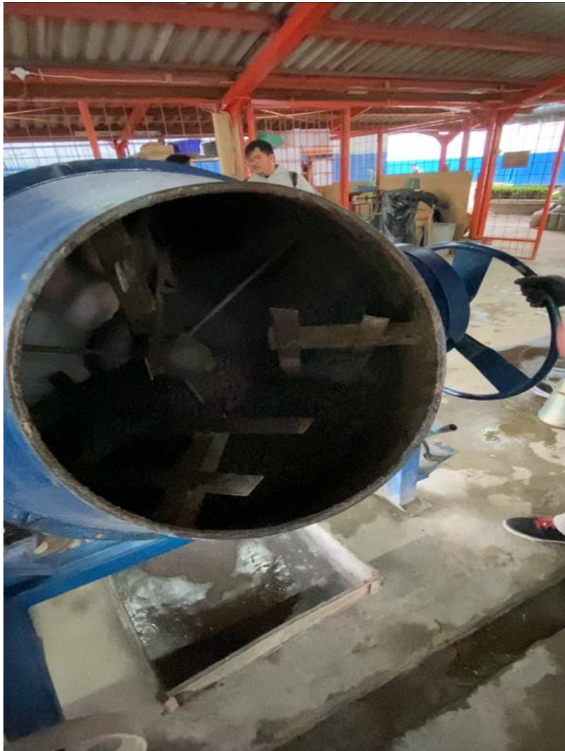
Lampiran 3 Pengecoran Campuran Beton Growblock
