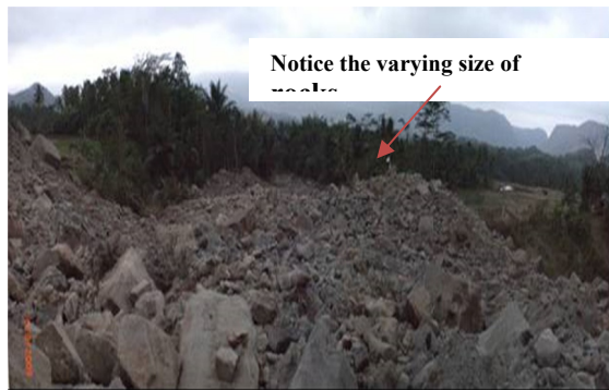
Fig. 12. Rockfall debris ( Rahardjo 6 Sept 09)
