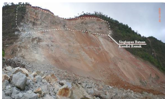
Fig. 13 Jointed rock and fractured rock exposed at the crown of rockfall
