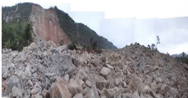
Fig. 7. The rockfall at Cikangkareng
