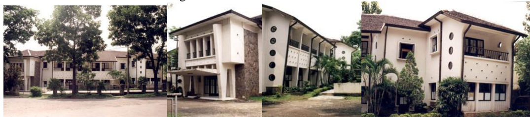
Fig. 3 Documentation of BPH Building Source: (Amelita, 2012)
