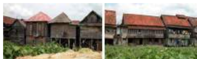
Figure 10. House Stage Warehouse.
